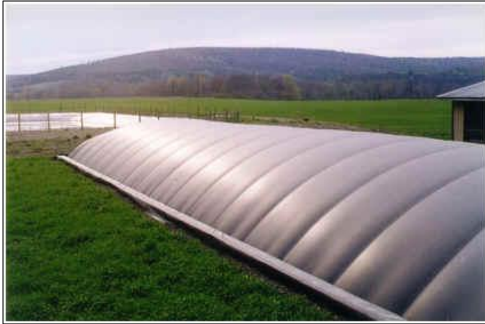
Plug Flow Digester (Source: http://www.plugflowdigester.com/ )
