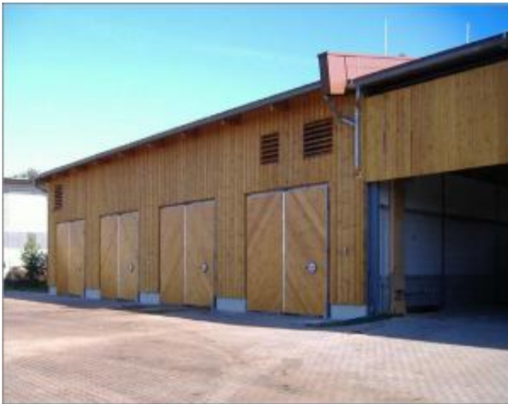
Figure 6: Dry Fermentation Digester
