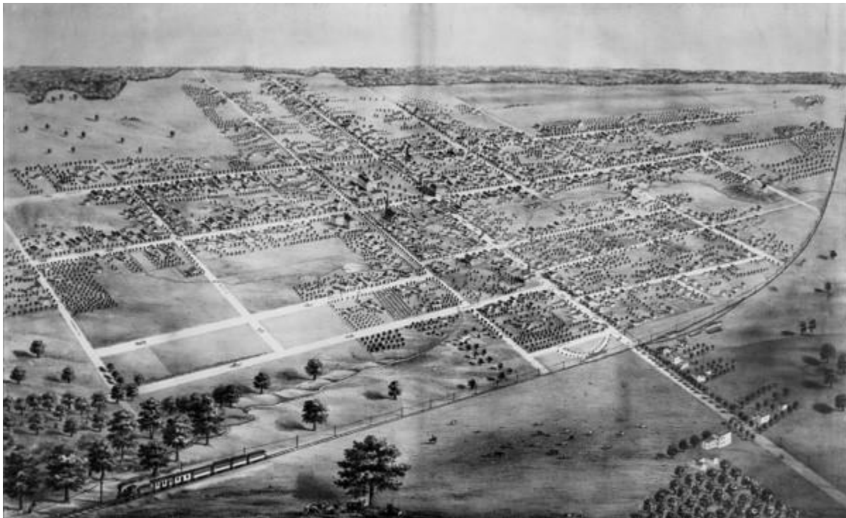
1868 View of the Town of Oberlin, Ohio. Photo Courtesy of Oberlin College Archives.
