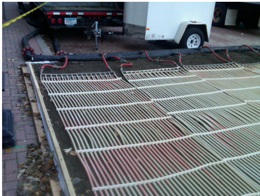
Figure 4.3. In-bed Heating – PEX Tubing
