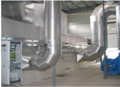
Figure 4.5. Belt enclosure with heated air circulation
