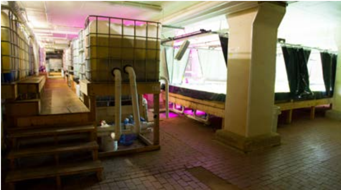
The aquaponic system at the Plant, located in the basement of the facility, features a series of fish tanks producing tilapia or perch. The fish effluent is circulated through growing beds to raise a variety of vegetables. The bio-digester for the Plant will generate electricity for indoor grow lights and heat for the aquaculture tanks.
